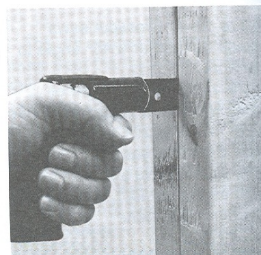
Figure 11-11. A nail saw is used to cut nails so that framing members can be more easily parted.
